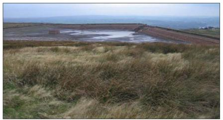
Figure 5. Reservoir emptied, notch cutting works commencing
