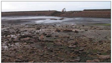
Figure 4. Reservoir emptied, notch cutting works commencing
